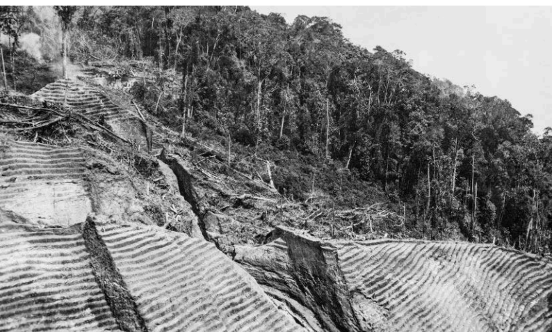
Figure 6. In the late 1920s, mining operations at Chivor under Rainier still used the traditional open-cast step-cutting technique. Terraces or steps were cut into the surface of the extremely steep mountain slopes, and the debris was washed away via water previously collected in tanks. Photo from the Peter W. Rainier collection; courtesy of GIA.
